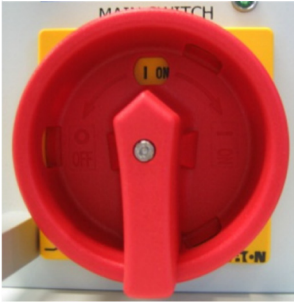
總開關 ( MAIN SWITCH )
